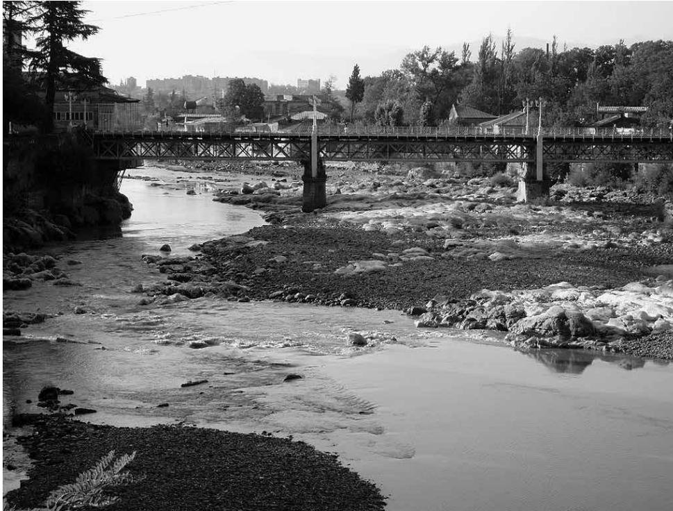
**Photo 1.** Erosive bed of the Rioni river on the reach of Kutaisi city, below the Rioni HPP water barrage. Photography taken by the author on 30.08.2007.
